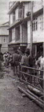
Landslide had occurred near Sikkim Rehabilitation Centre at Mile 32, which brought the national highway traffic to a
